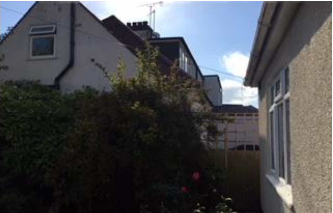
Flank wall of No.25 The Glen
