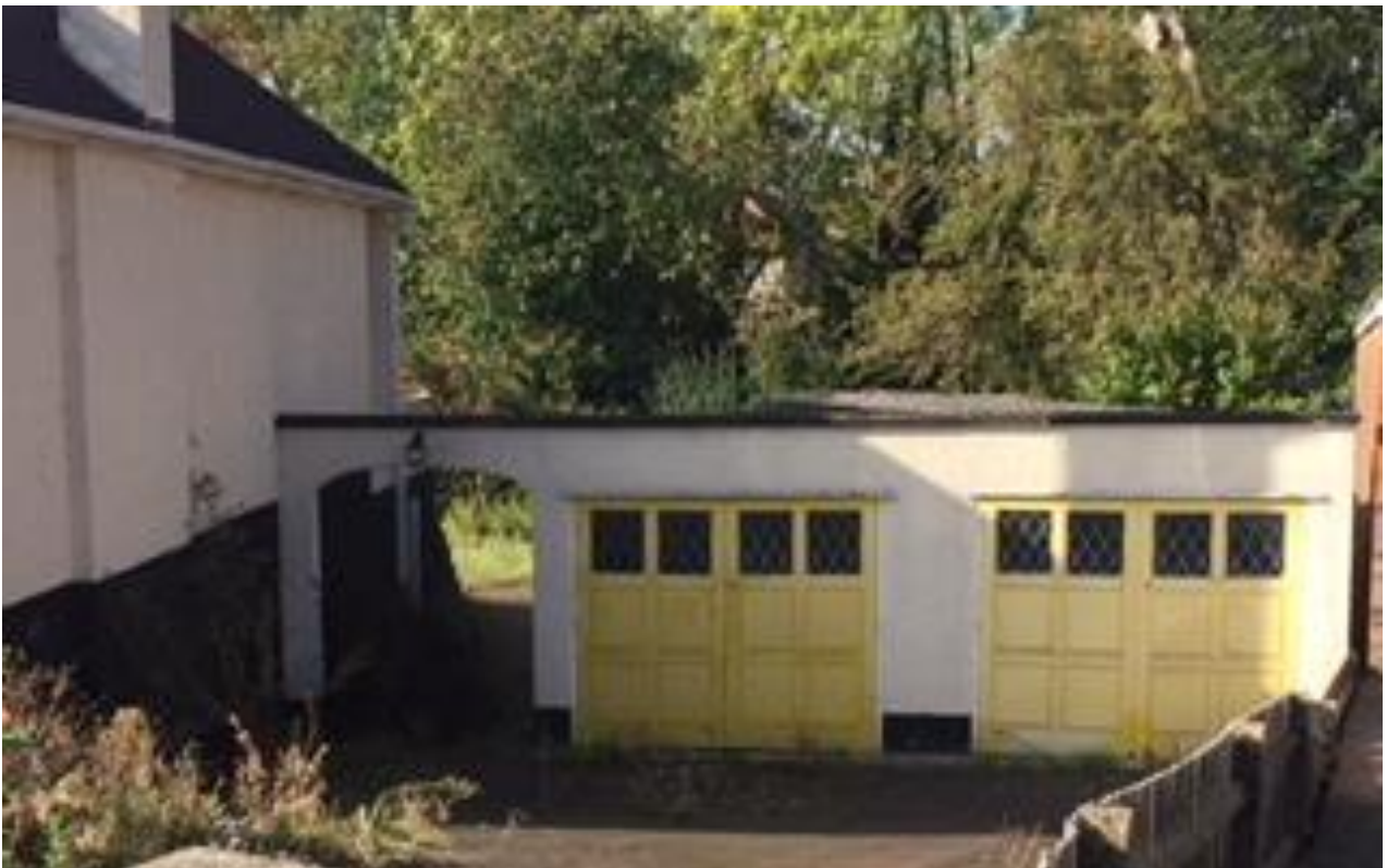
Existing garage at host dwelling
