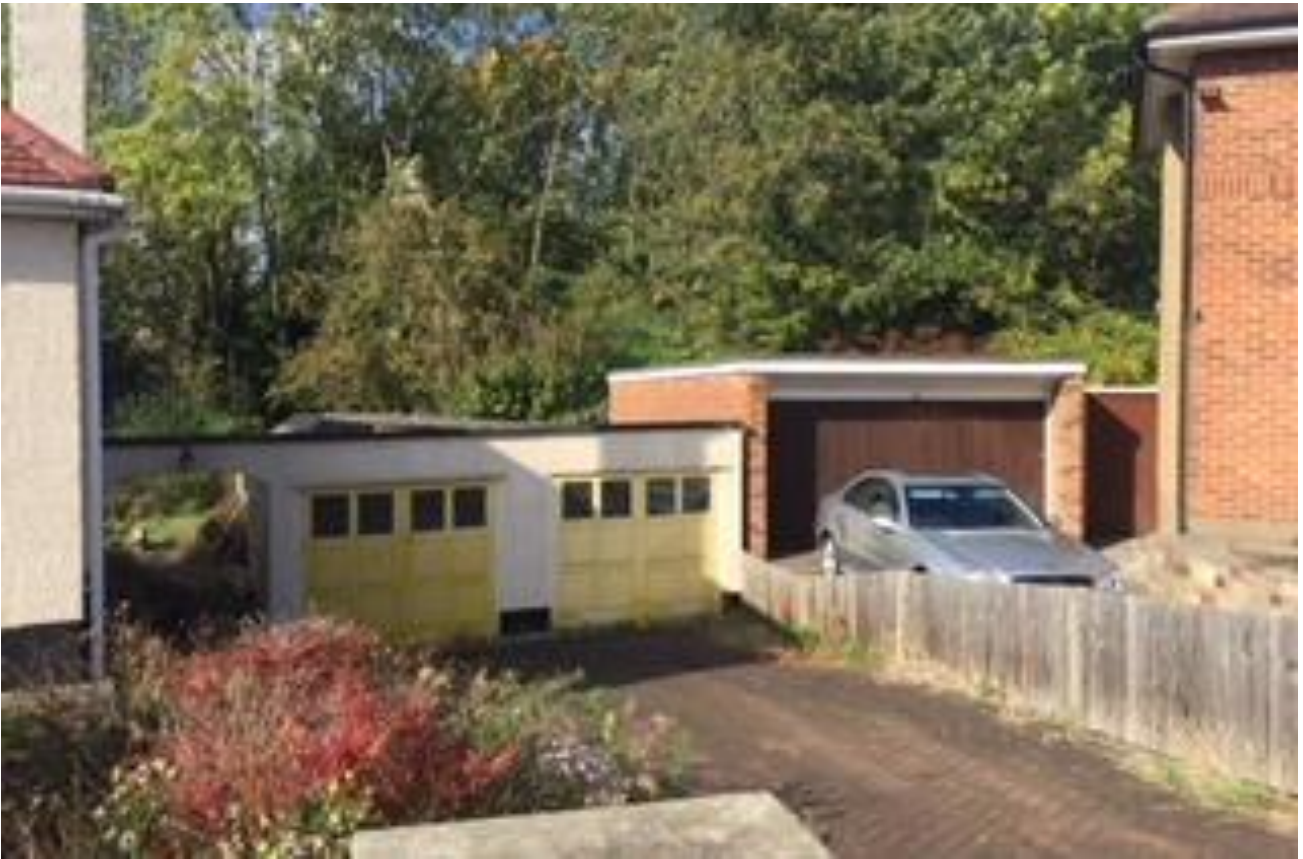
Existing garage at host dwelling, flank wall of No.29 The Glen
