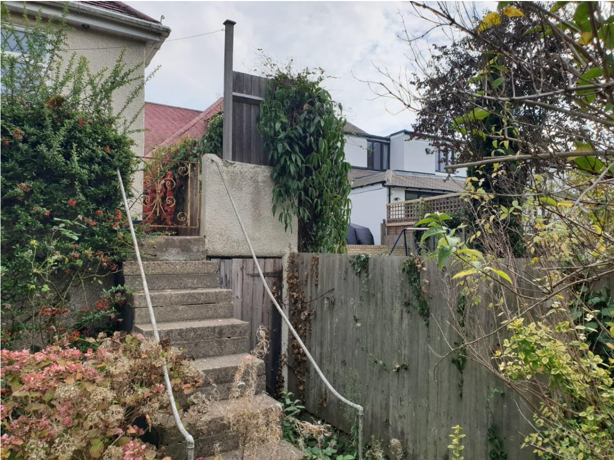
Rear elevation of No.29 The Glen
